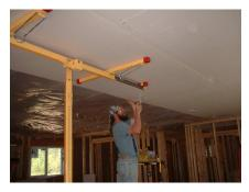
We have completed the vapor barrier that covers the fiber-glass insulation, ceiling drywall,
